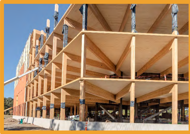
Construction of First Tech Credit Union, Portland Photo credit: Mike Brewington
