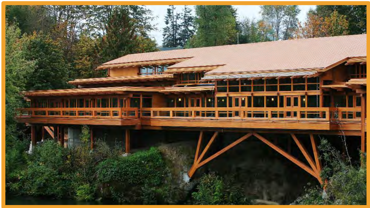
Tseshaht Tribal Multiplex and Health Centre, Port Alberni, B.C. | Photo credit: Lubor Trubka Architects
